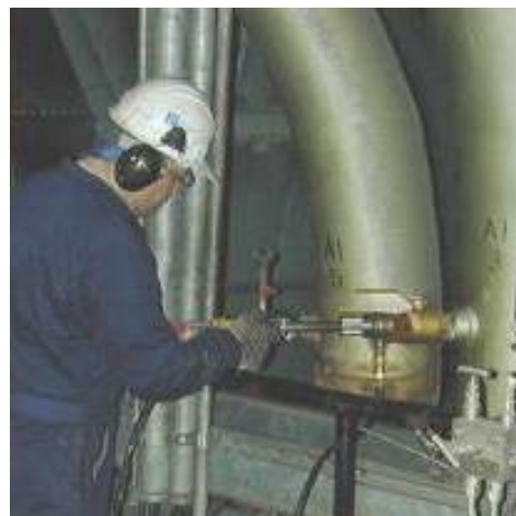
ASME PTC 4.2 sampling in a coal pipe
