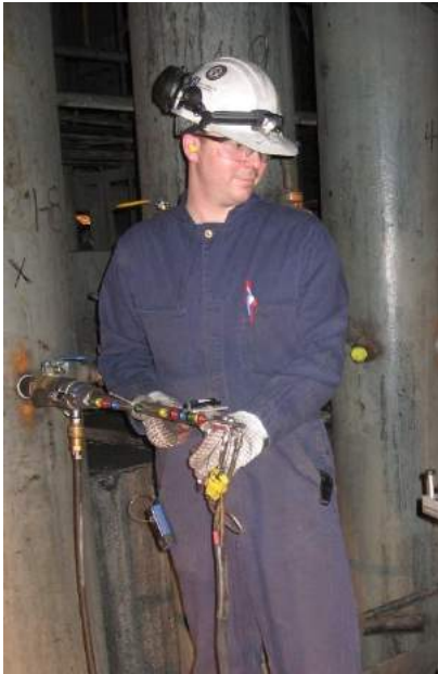
Velocity testing in a coal piping system
