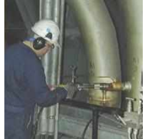
ISO 9931 sampling in a coal piping system
