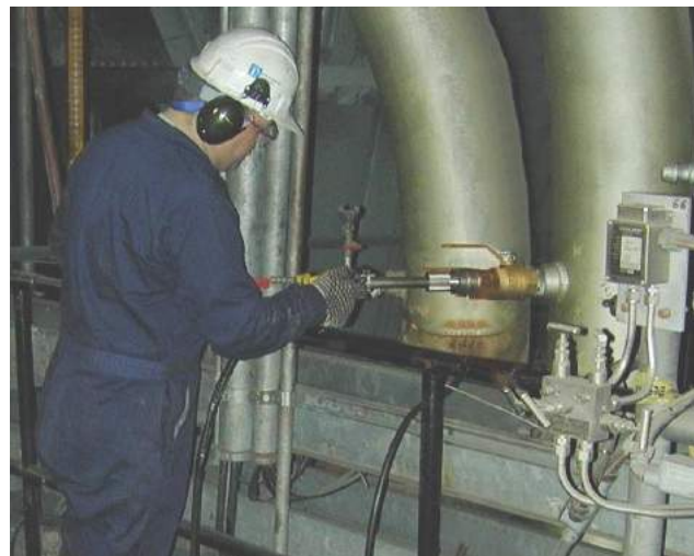
IsoAsh sampling in a piping system
