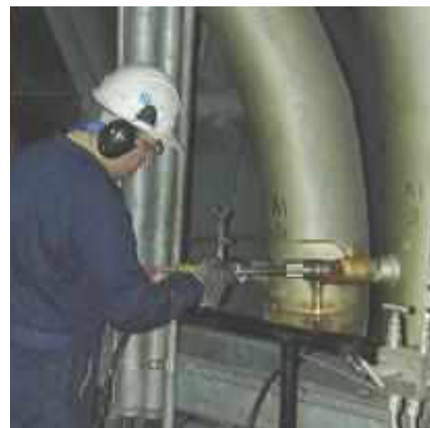
ASME PTC 4.2 sampling in a coal pipe
