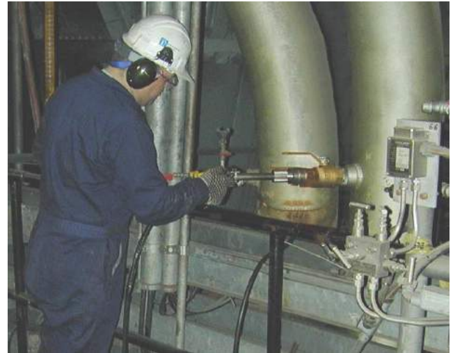
IsoAsh sampling in a piping system
